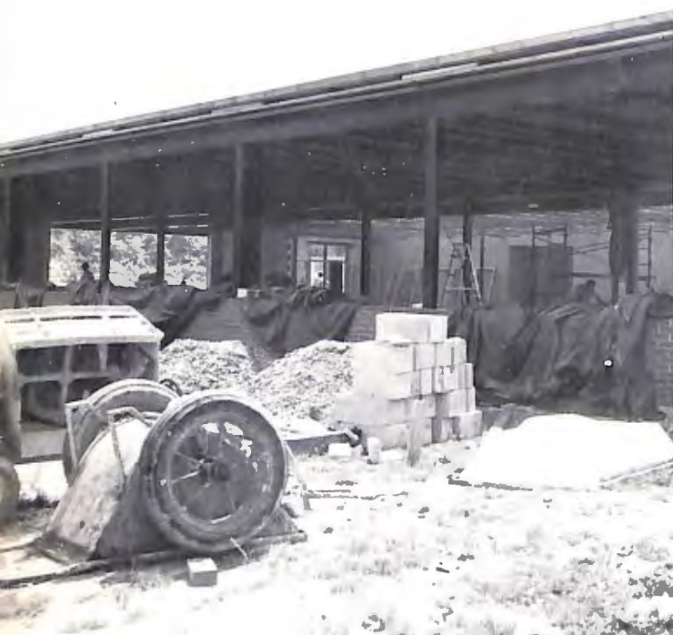
Construction of a new addition brings six needed rooms and many lockers for the people who shared.
