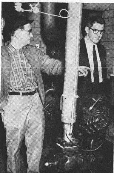
J. T. McLain, air conditioning engineer, and Mr. Buchanan, right, discuss heat pump equipment in the penthouse in the General Office Building.
