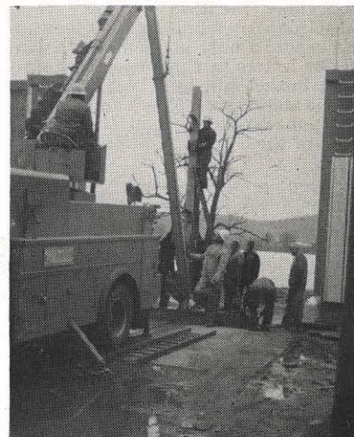
The Point Pleasant line crew places steel for the 4th Street flood gate. Called into emergency service, the new truck reduced the time for installing the gate by several hours. The crew also installed the gate at Tu-Endei-Wei Park.
