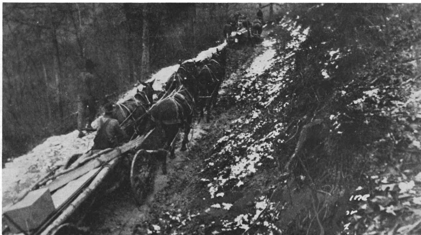
"The crews used teams of oxen to snake poles up the hillside." This picture was made in 1924 during construction of the St. Albans-Logan line.
