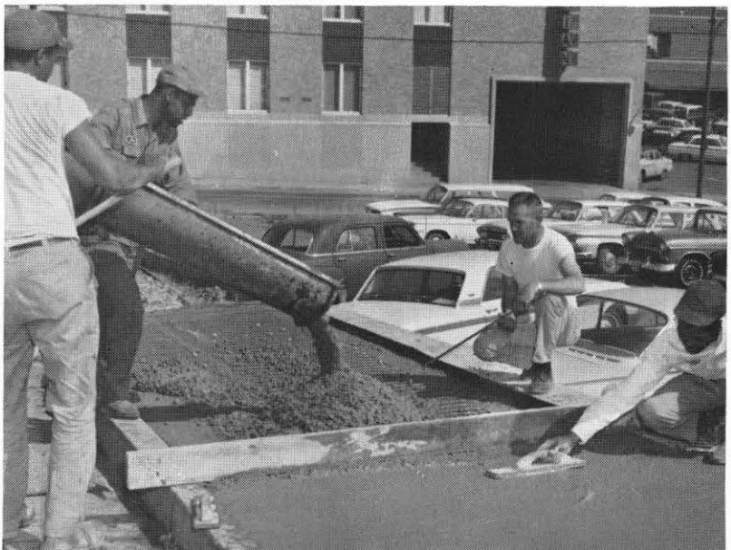
If you sell electric, melt electric. So says Appalachian, which last month completed the installation of 3,000 square feet electric snow-melting cable in the sidewalk around the company parking lot just to the rear of the main office building. This job is the third in the immediate vicinity of the building: one being around the building's addition, the other by the company's other parking lot.
