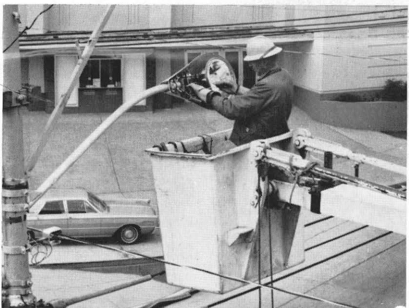
Just outside the window of Appalachian's Virginia Street office, H. M. Bailey installs one of the 41 21,000-lumen mercury vapor lights going up on that thoroughfare. The lighting program calls for the removal and replacement of a total of 69 old incandescent lamps.
