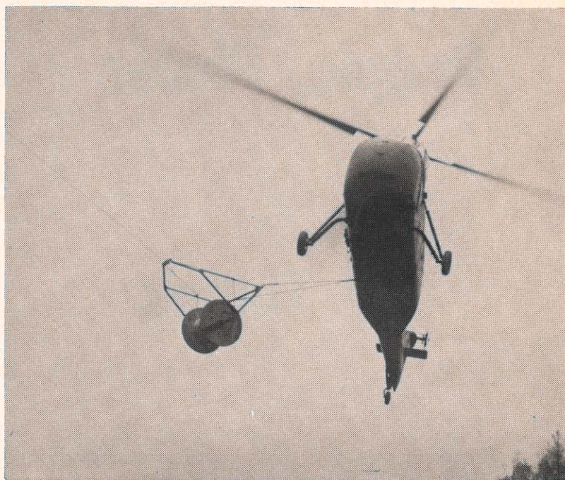
Helicopter carefully feeds out wire in the rugged Williamson area.
