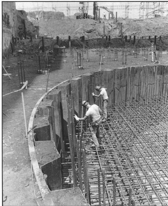
Workers ready the ring or support pad where the combustor vessel will be placed.
